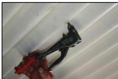
The underside laps of the panels need to be fixed at 300mm centres using pop rivets. The rivet should be placed just off to the side of the rib towards the lap. All holes for rivets will need to be pre-drilled.
