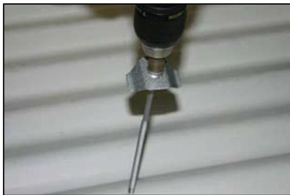
Continue to lay out the panels, constantly checking that they are parallel as you go. Continue to screw down each panel into the support structure.
