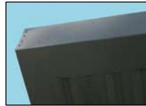
For the capping along the run of the roof, rivet at 300mm centres, aligning with the stitching screws. Silicone the corner capping joins top, side, and bottom to ensure no leaking. Use only neutral cure silicon. All holes for rivets will need to be pre-drilled.
